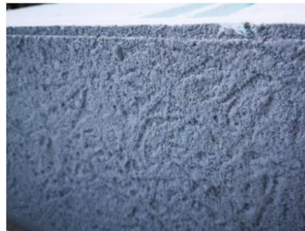
Figure 5 - Primary protective finish
